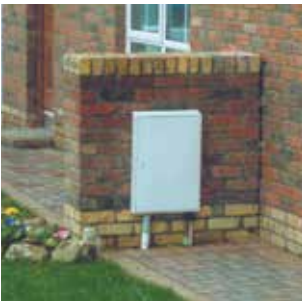
Domestic meter box
