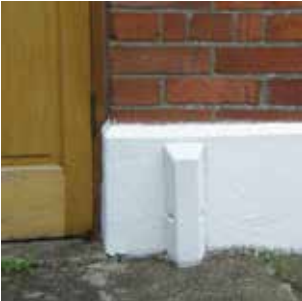
Service riser cover
